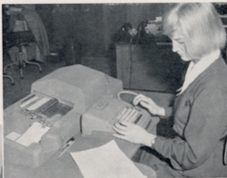
Key Punch punches original holes. Cards are checked by Verifier and arranged by Sorter
