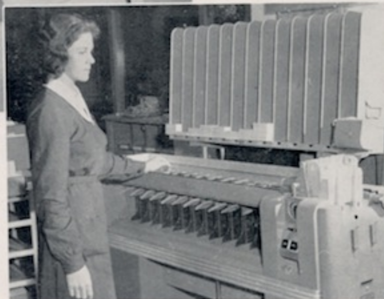
Key Punch punches original holes. Cards are checked by Verifier and arranged by Sorter
