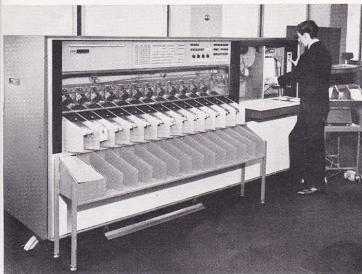
● THIS sorter reader at The Reserve Bank, Melbourne, "reads" magnetic ink at the rate of 1600 cheques a minute.
