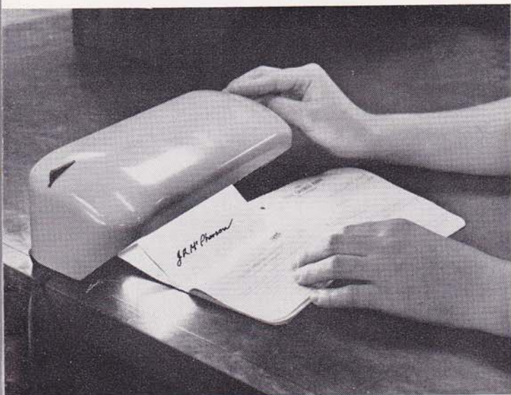
A close-up of the insert shows how the "black light" brings up the latent signature.
