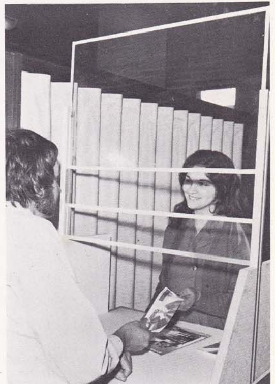
BANDIT BARRIER: This is one of two installations being tested — with the object of preventing bandits from vaulting tellers' and inquiry counters.
